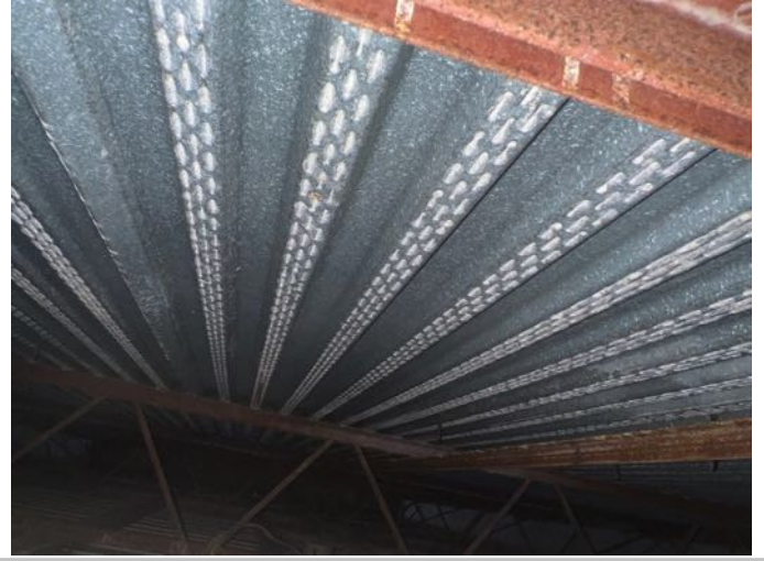
corrugated concrete deck form
